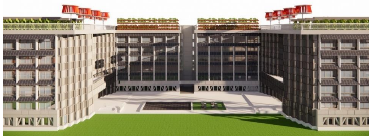
Figure 20: south new façade.
