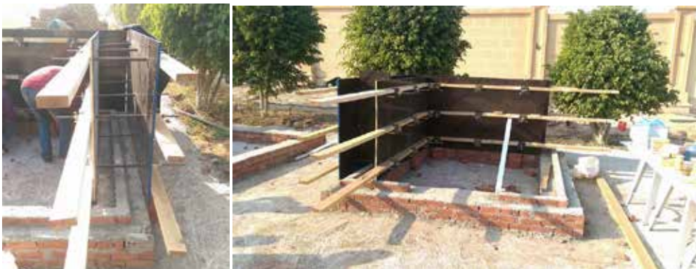
Fig. 10. Wooden Formwork for constructing Rammed Earth Wall.
