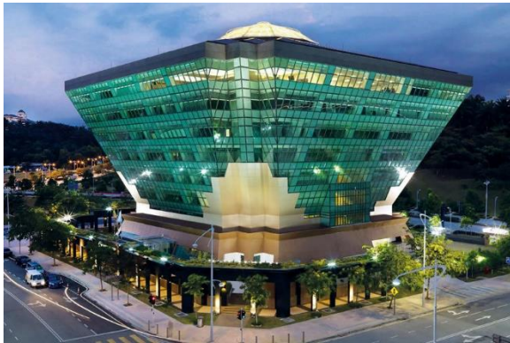
Figure 1. Self-shading inverted pyramidal form of the ST Diamond Building, Putrajaya, Malaysia (Source: M. Boubekri, 2014).
