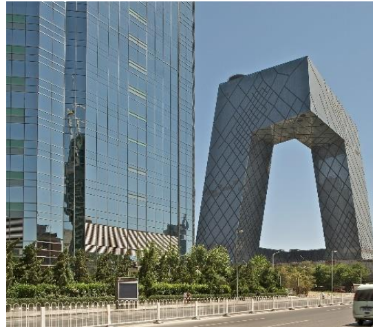
Fig. 10 CCTV Headquarters in Beijing. [15]
