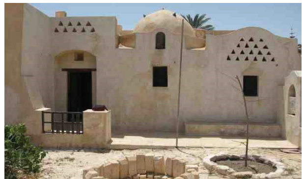
Figure 12. The use of local lime stone in Hassan Fathy's Sidi Krir house
