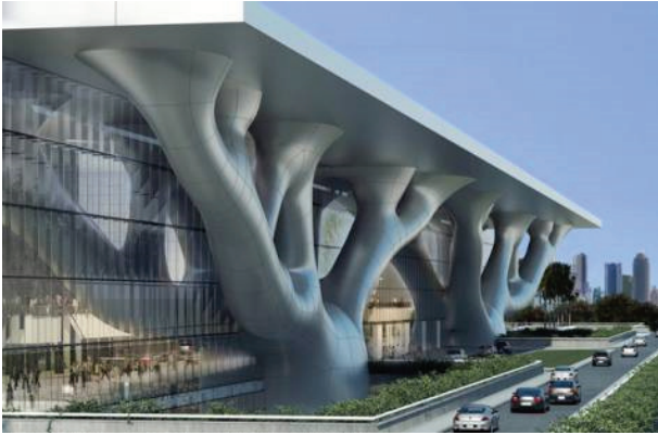
Figure 1. Qatar National Convention Centre
