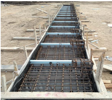
Fig. 3 Preparation form work and reinforcement.
