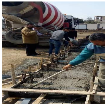
Fig. 4 Concrete casting-in-situ.
