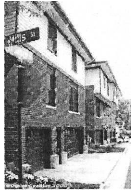
Figure 8 Carefully graded site
