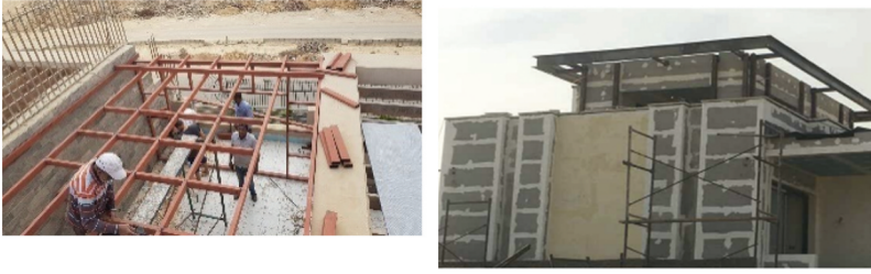
Figure 4. Marmox board construction in a residential building.
