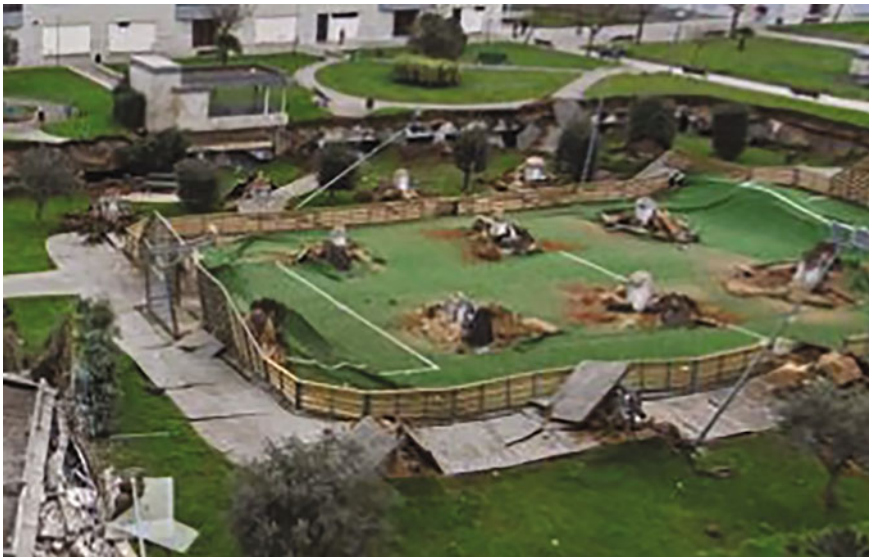
Fig. 14.1 Parking garage atop a playground collapsed (Deifalla 2022)
