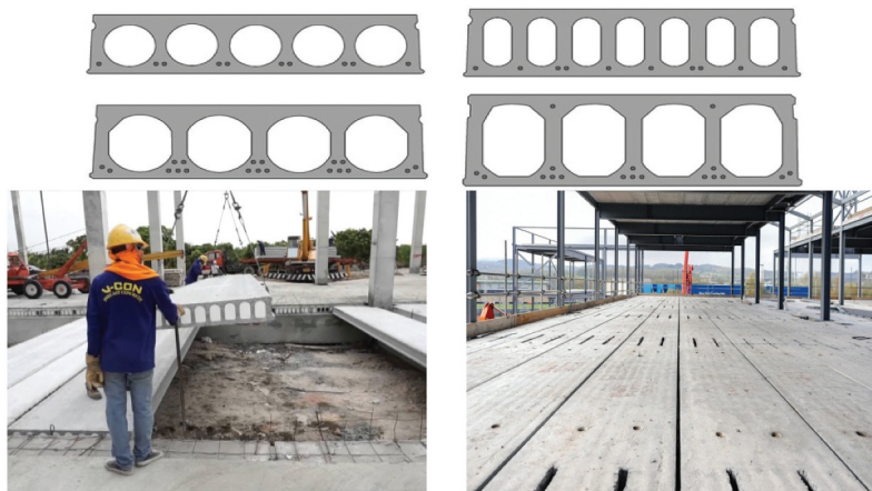
Figure 2. Types of hollow-core flooring systems.
