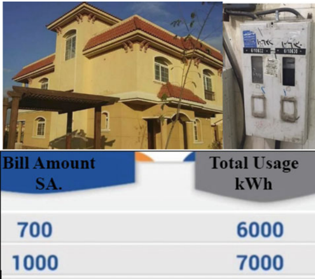
Fig. 10 The actual validated villa in Al Riyadh and the installed electricity meter
