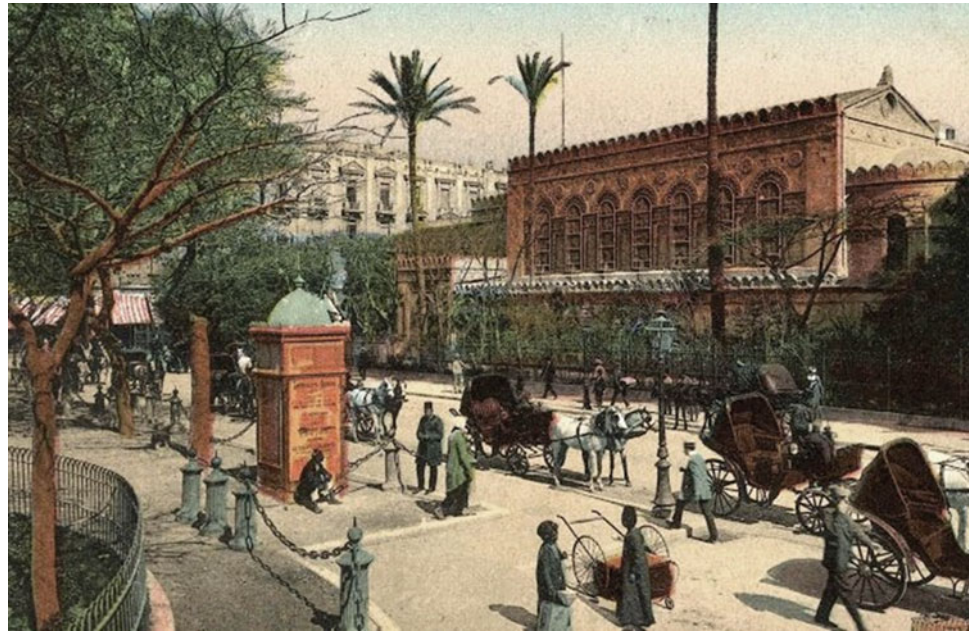
Fig. 7 St. Marks church. Source Humphreys (2019)
