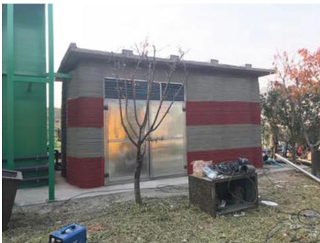
Fig. 4 3D printed concrete sewage treatment equipment room
