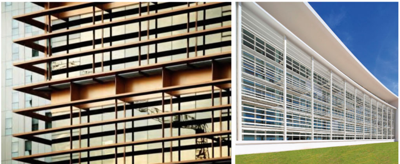
Fig. 3 The horizontal shading devices within the Head Office constructing of the telecommunications market commission (CMT), Barcelona, Spain
