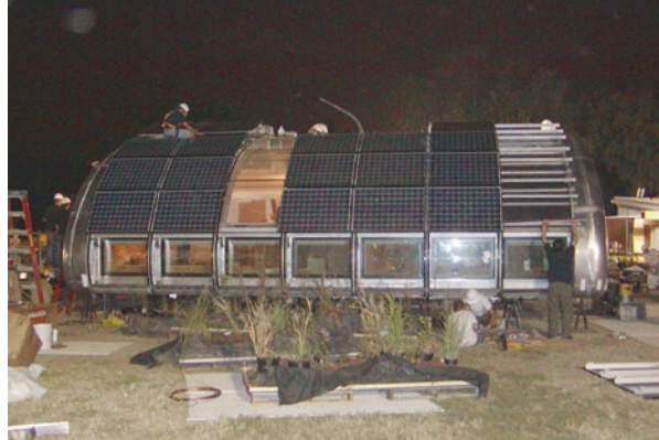
Fig. 14.9 The Michigan Solar House (MiSo) during its construction (D. Oktay Archive)
