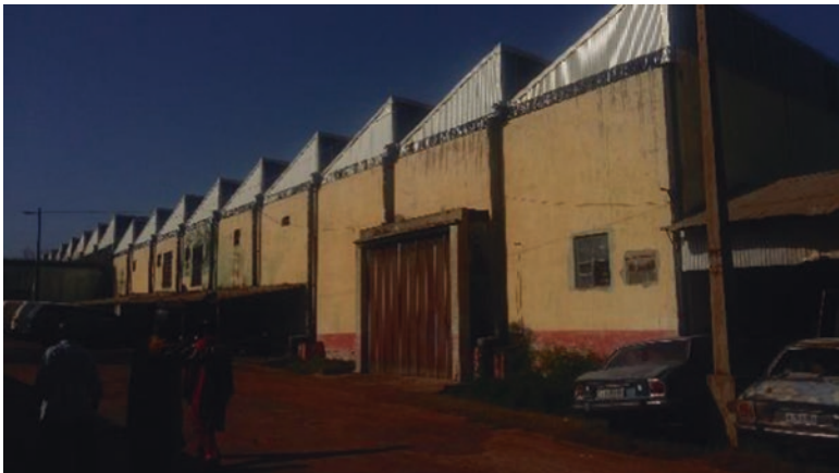
Plate 20.5 Façade at Kaduna textile limited (Source: Author's field work)
