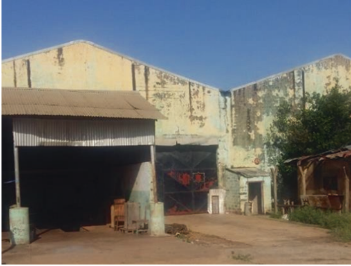
Plate 20.10 Factory building with rectangular plan and gable roof (Source: Author's field work)
