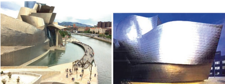
Fig. 14.1 (a, b) An example of shape-oriented building designed with the intention of creating a focal point through its form: The Guggenheim Museum Bilbao, by Frank Gehry (D. Oktay Archive)
