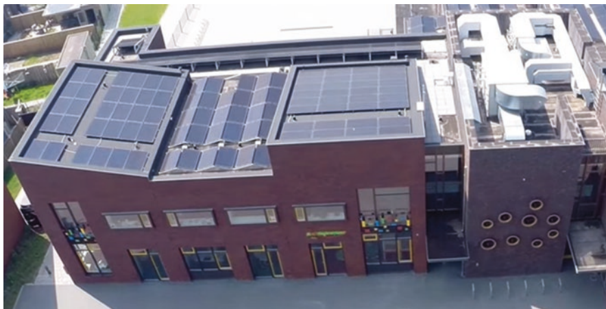
Fig. 15.4 Overview energy generation by PV panels of school 1 [9]
