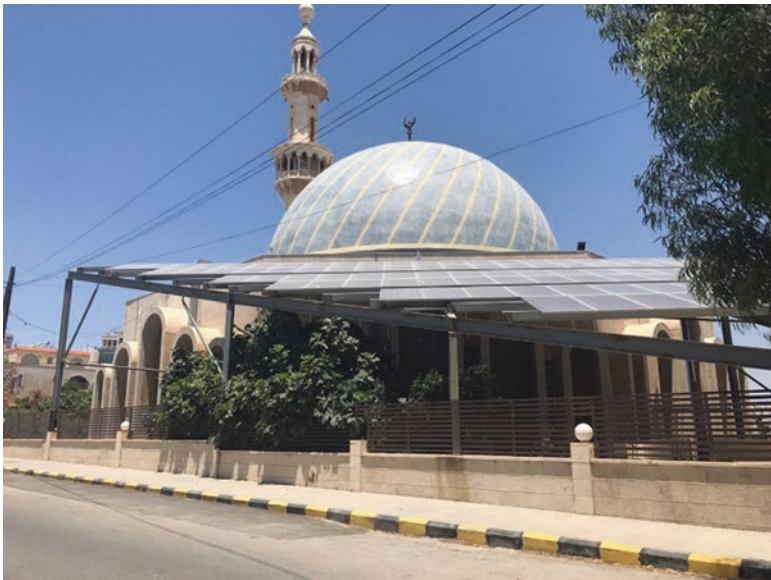
Image 48.2 A mosque with installed photovoltaic panels. Photo Credit: Zaid Marji
