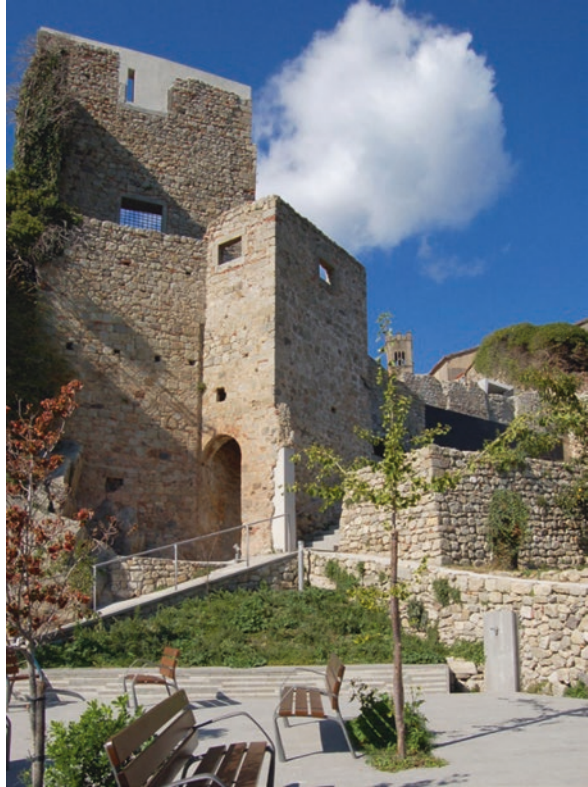
Fig. 37.7 Santa Fiora Village in Tuscany. View of rehabilitation actions of courtyards, towers, walls and house buildings, according to the valorization of environmental performance
