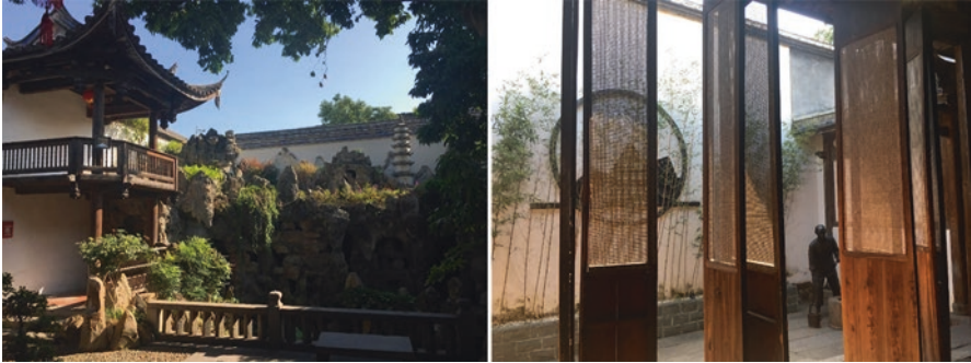
Fig. 2.5 Left: the lavish indoor garden for the family use, with its environmental function of providing outdoor shaded areas. Right: the handcrafted wooden screens to provide shelter from the hot summer heat awhile allowing for natural ventilation. Photos: author's personal collection
