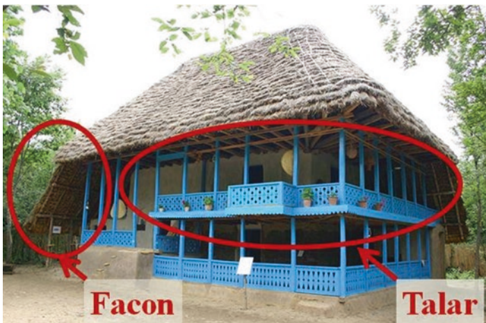
Fig. 7.16 Integrated balconies and Facon (west side)—Moradi house (Taleghani 2011a, b)
