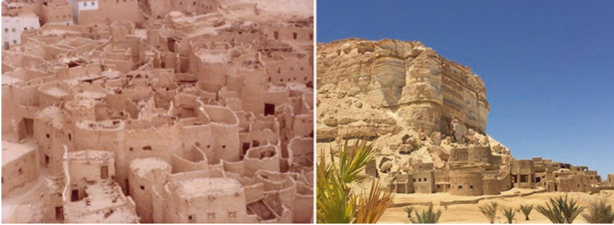
Fig. 2.10 Left the ruins of Shali village-Siwa, Egypt. The compact urban defensive configuration with their circular observatory towers built from the local materials creating the Kershef construction method. Photo courtesy: Prof.Hatem Altaweel. Right the vernacular contemporary interpretation in Hotel Adrer Amelal, Siwa, Egypt. The creation of the exotic encounter with local culture. Photo courtesy: Prof.Heba AbulFadl, July 2016
