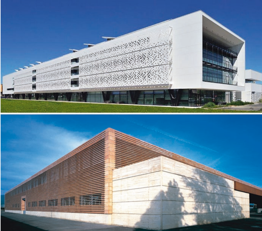
Fig. 12.25 Double envelope and ventilated facades realised with different materials. Metallic and brick shading devices
