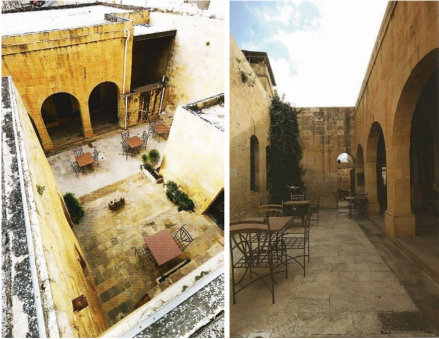
Fig. 8.7 Courtyard walls help to create shaded areas and enhance the natural ventilation and lighting (Touqan house). Source: Architecture heritage in As-Salt city, Jordan (As-Salt City Development Projects Unit 2016)
