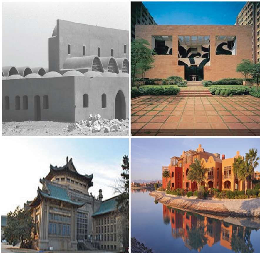
Fig. 2.1 Top left: Hassan Fathi New Baris Village; beautiful but expensive to build vaults and domes, considered crucial for the thermal and daylight performance on the buildings (courtesy, Google images). Top right: Charles Correa interpretation of the Indian vernacular symbolism in the British Consulate, Delhi, India (courtesy, Google images). Bottom left: F.H. Kales, Wuhan University old Library with its distinctive and expensive decorative blue vernacular construction and materials of tiles and timber decorative elements. Bottom right; Michael Graves, Elgouna Tourist Village, Red Sea, Egypt, a speculative development of five-star hotels and separate vernacular style villas exist for the enjoyment of the rich. ElGouna resort in Egypt designed by the international architect Michael Graves, as a speculative development that, earned from the architecture of Egyptian architect and advocate of the Nubian architecture style as architecture for the poor turns into this speculative ecotourism attraction where five-star hotels and separate vernacular style villas exist for the enjoyment of the rich at a premium
