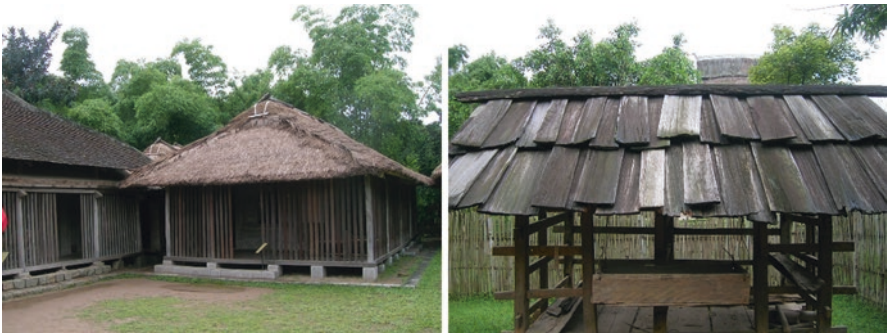
Fig. 16.3 Vernacular architecture defined by roofs in Hanoi
