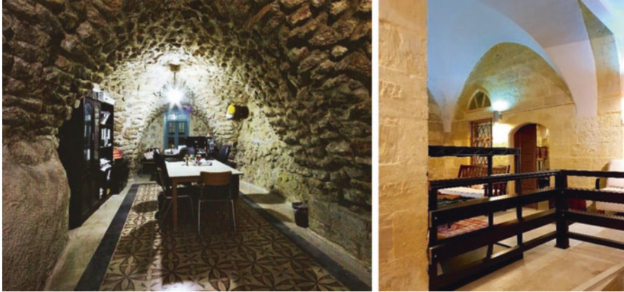
Fig. 8.13 Construction system (vault and cross-vaulted ceiling). Source: Architecture heritage in As-Salt city, Jordan (As-Salt City Development Projects Unit 2016)
