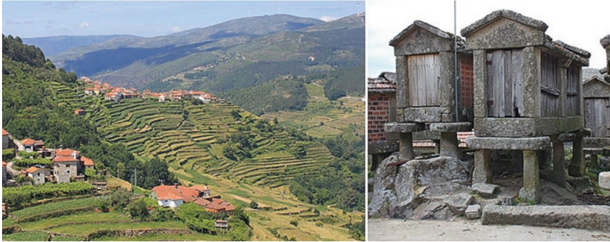
Fig. 4.4 Terraces in Valley of Vez between Padrão and Porta Cova, and Granaries of Padrão (credit: Barros et al. 2016)
