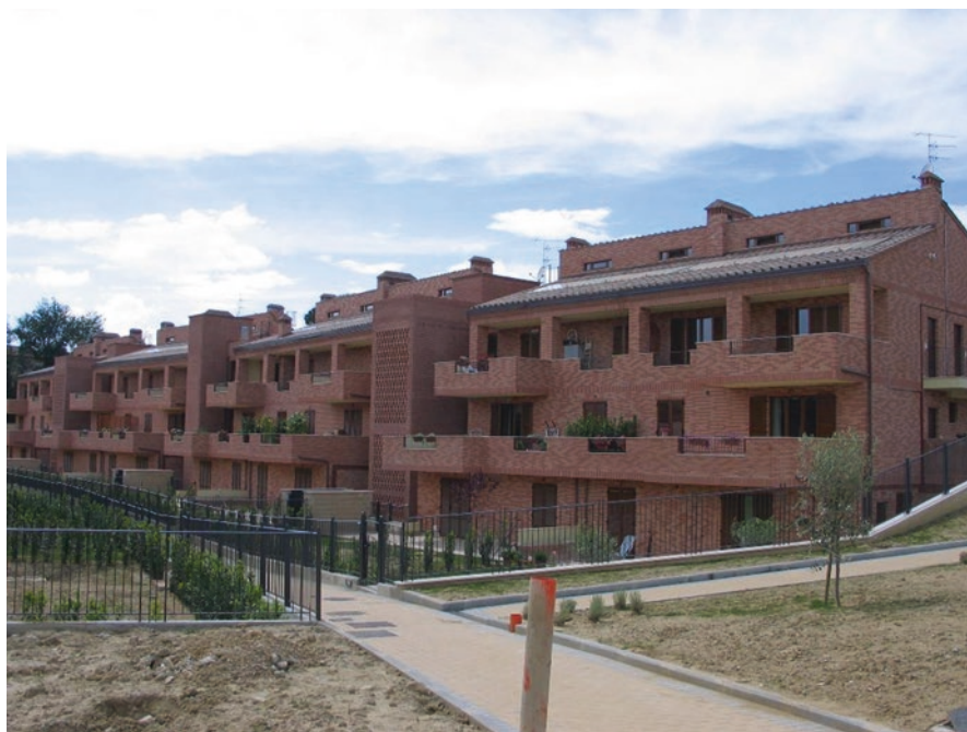
Fig. 12.22 Modern apartment house near Siena, with traditional brick cladding and the replica of brick grid as sun blind for the staircase. PV panels integrated into the roof, and not superposed to it. Large terraces protect windows of lower floor from direct sun radiation. (Project in Castelnuovo Berardenga, by Marco Sala Associated)
