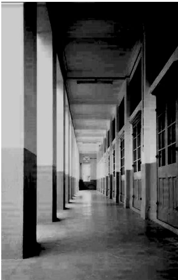
Fig. 14.6 Classroom block in Victoria Institution
