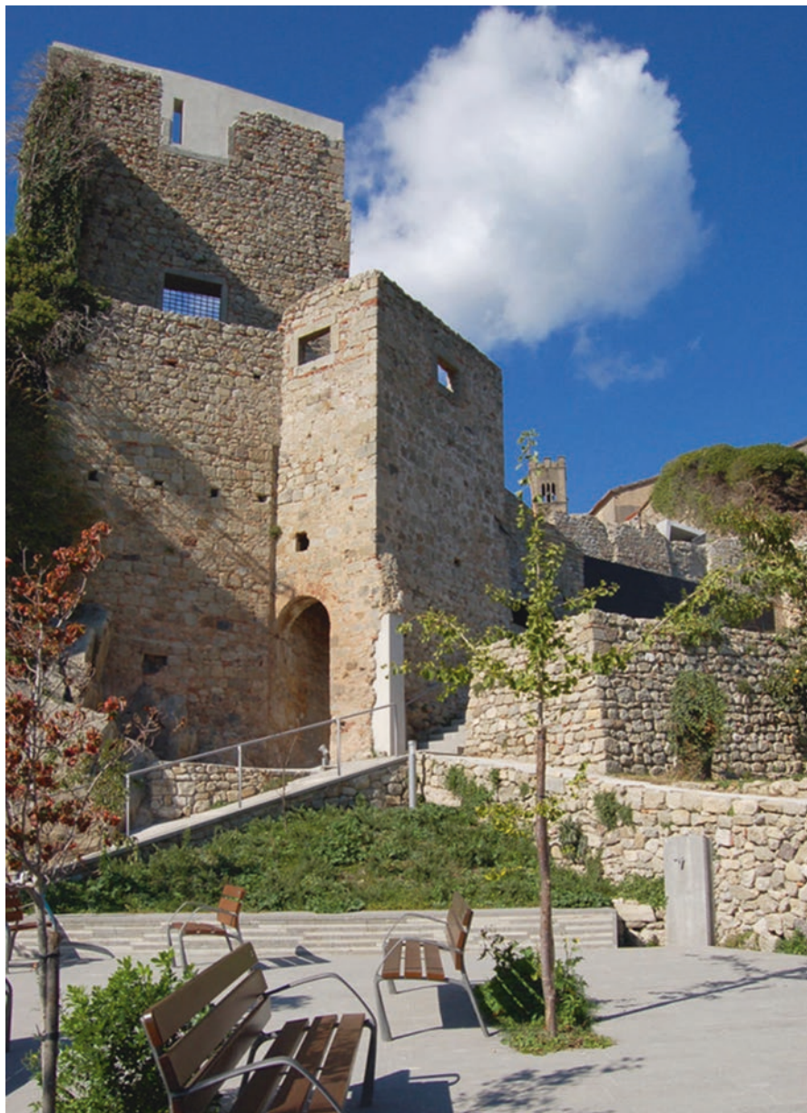
Fig. 12.15 Santa Fiora village in Tuscany. View of rehabilitation actions of courtyards, towers, walls and house buildings, according to the valorisation of environmental performance
