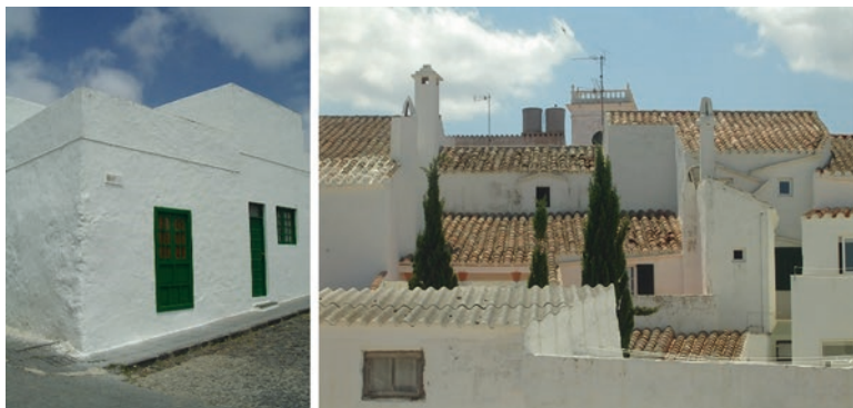
Fig. 16.13 Flat roofs in Lanzarote and pitched roofs with Arabic tiles in Menorca
