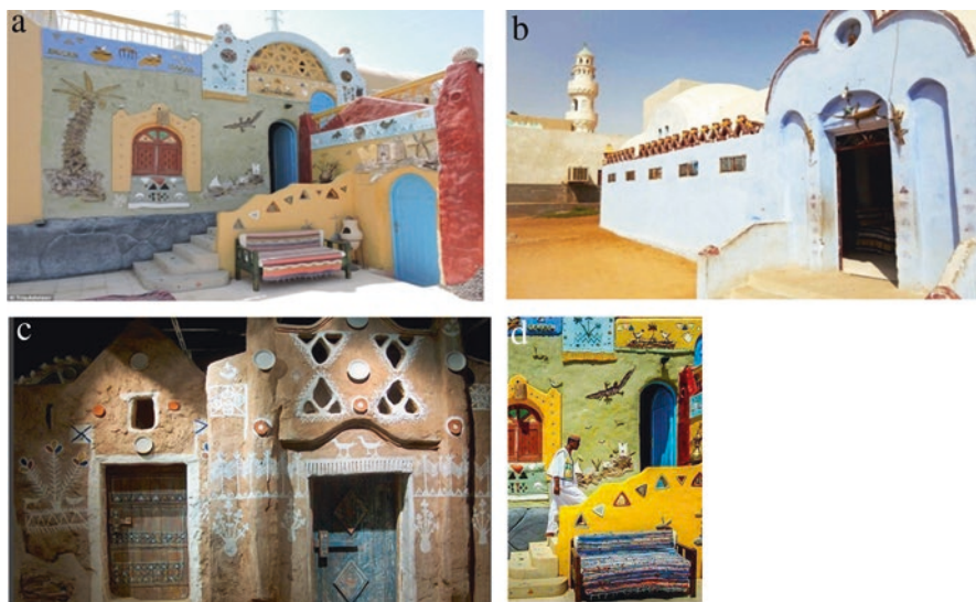
Fig. 15.12 Old Nubian architecture, Upper Egypt. (a) Vivid colours and decorations in guest house http://www.dailymail.co.uk/travel/travel_news/article-3341353/Anakato-Nubian-guest-house-oasis-colour-Egyptian-desert.html . (b) Minimal openings in exterior elevation. https://www.egypt-toursplus.com/nubian-village/ . (c) Small triangular openings in a Nubian house. http://looklex.com/egypt/aswan12.htm
