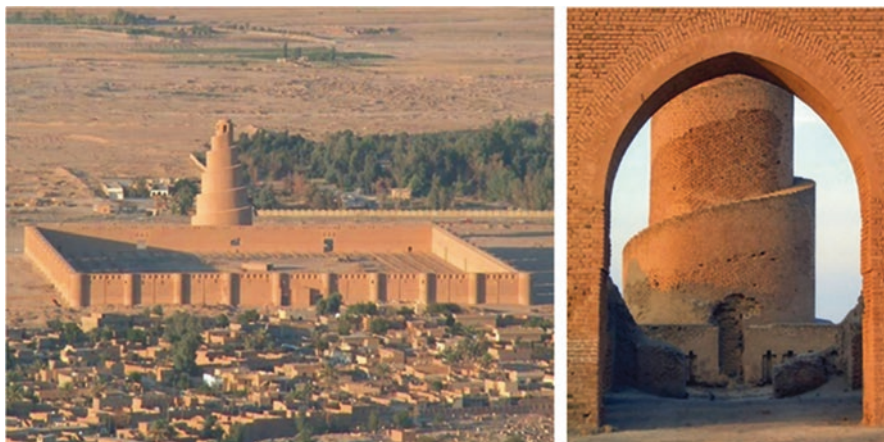
Fig. 10.4 The general view and the door of Great Mosque of Samarra
