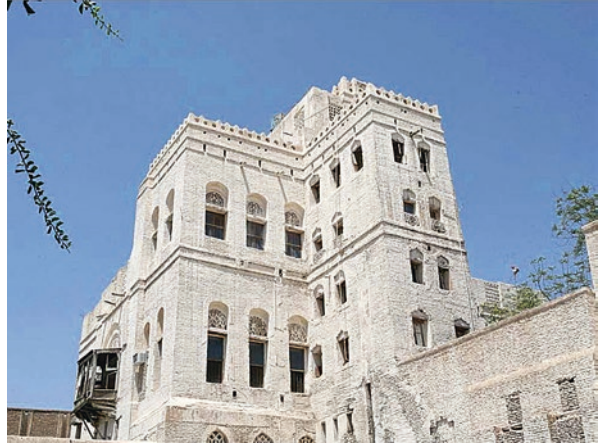
Fig. 3.14 Minimizing heat gain via white color of the building's envelope as demonstrated by the traditional architecture of Zebid, Yemen (ERYJ 2016)
