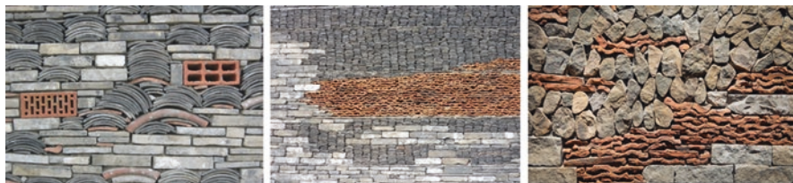
Fig. 10.26 Details of the external wall made with the rubble coming from the destroyed areas of the city to ensure memory and continuity with the recent history. Reference: Wang Shu—Ningbo History Museum
