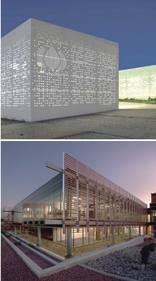
Fig. 12.26 New concept design for shading and translation of vernacular architecture to control direct solar radiation
