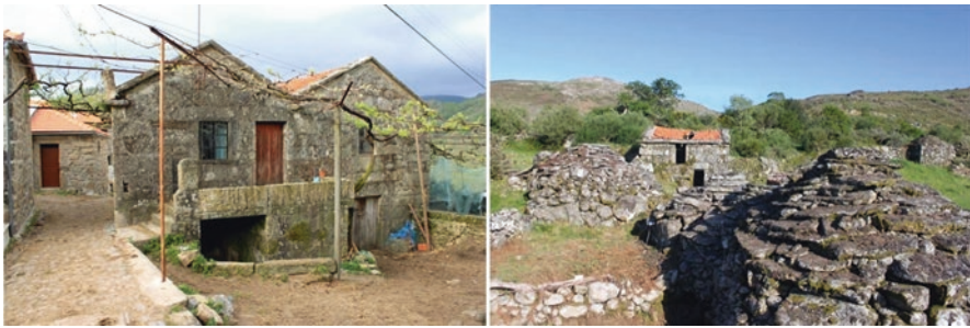
Fig. 4.5 Granite houses in Padrão's village, and houses and pastoral shelters constructed in corbelled dome structure at Gêmea's summer village (credit: Fernando Cerqueira Barros)
