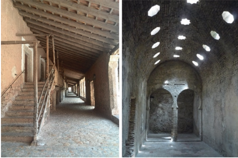
Fig. 16.4 Lintelled porch in Mallorca and vaulted coverage in the Arabic Baths of Granada
