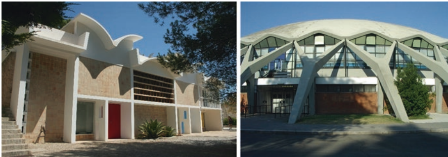
Fig. 16.15 Use of concrete roofs in Joan Miró studio, Palma de Mallorca and Palazzetto dello Sport, Roma
