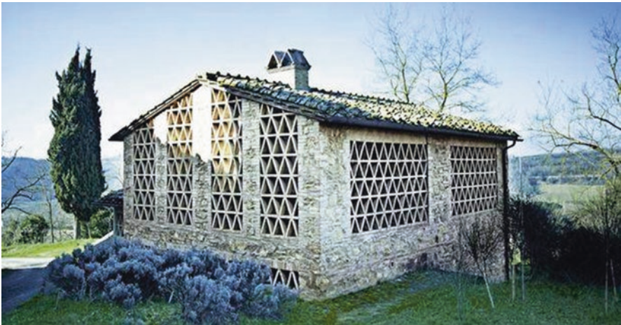
Fig. 12.19 Typical fenile , the traditional rural building in Tuscany, with stone structure and brick grid to allow ventilation
