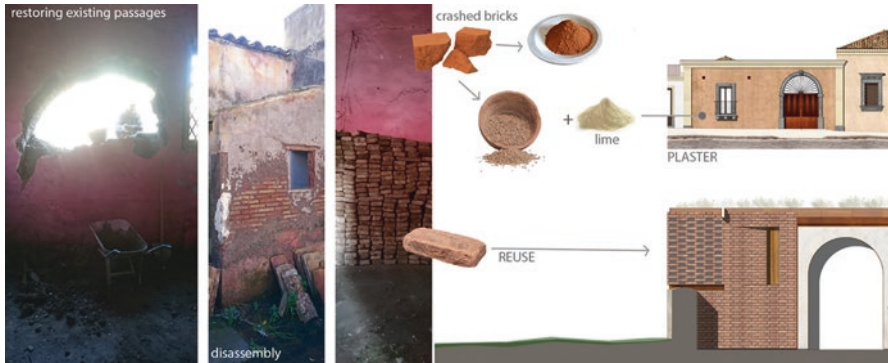
Fig. 13.10 Materials provided by disassembly of existing structures and by opening existing passages have been sorted for nature and condition. This material was reused for building the new service core and sorted for producing plaster to be used in the next project stage
