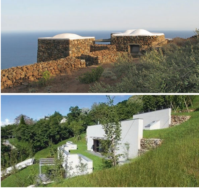
Fig. 12.9 The typical dammuso in the island of Pantelleria and a semi-hypogean in the countryside of Marostica
