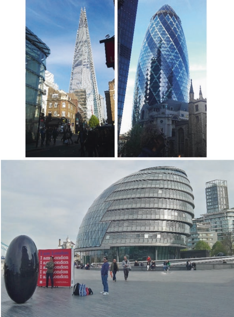
Fig. 16.19 Some examples of glass architecture where the boundaries between roof and façades are not defined; The Shard, 30 St Mary Axe and London City Hall
