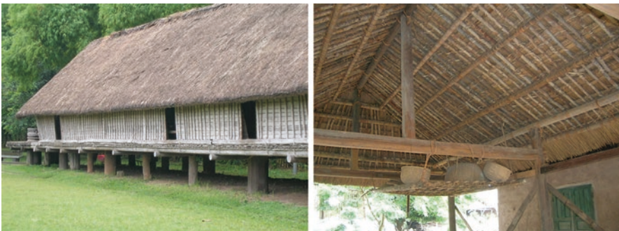
Fig. 16.11 Ventilated roofs in vernacular architecture of Hanoi, Vietnam
