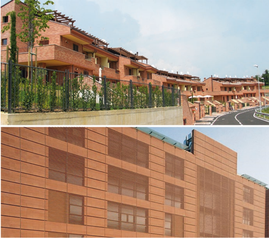
Fig. 12.23 Banca di Lodi, Italy. Brick solution of ventilated façade and shading devices, design by Renzo Piano
