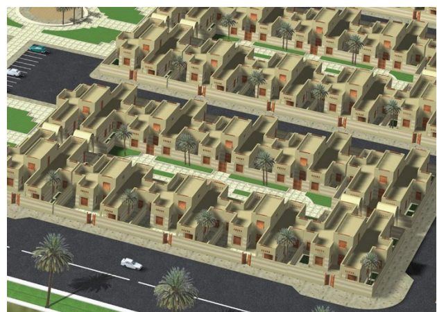
Figure 18. View of the residential cluster
